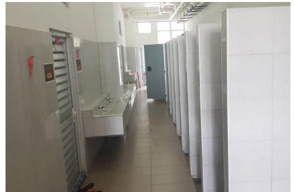
Bathroom – meets local regulations in terms of number of bathrooms in relation to number of occupants.
